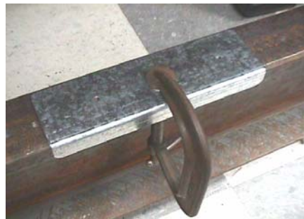
Fig 2.3 Drill guide in place
