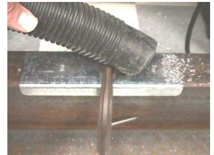
Fig 2.5 Clean up ALL debris
